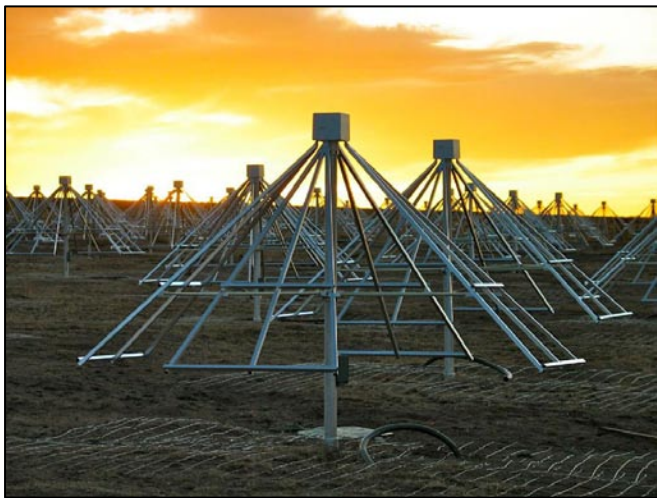
Multiple antennas of the LWA-1 station of the Long Wavelength Array in central New Mexico, photographed at sunset. Each antenna stands about 1.5 meters (5 feet) high and about 2.7 meters (9 feet) across the base. Image credit: LWA Project (at UNM)
