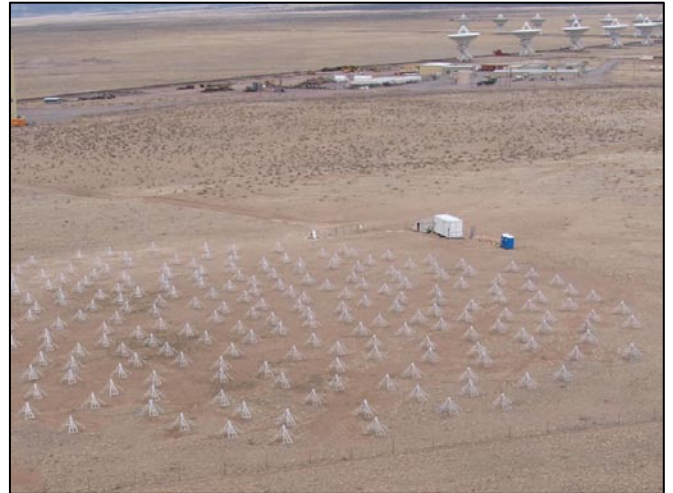
All 256 antennas of station LWA-1 of the Long Wavelength Array in Central New Mexico taken on April 1, 2010. The development of the Long Wavelength Array stations will proceed over several years. Construction for the second and third stations will begin in 2011. Eventually, the new telescope array will harness the power of more than 13,000 antennas. Image credit: LWA Project (at UNM)
