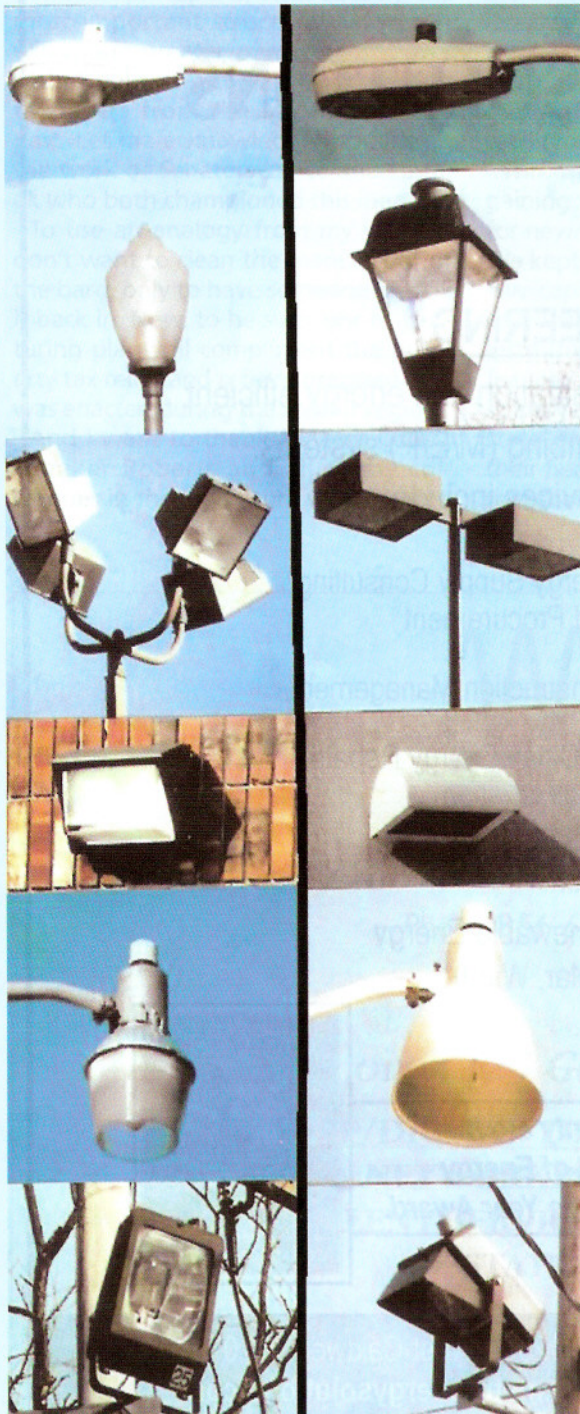
Non-cutoff, light pollution fixtures are shown on the left. The better alternatives are on the right.
